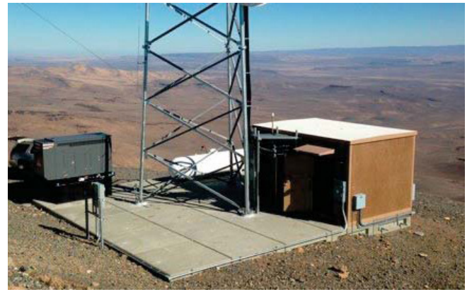
CELL BLOCKS Foundation with wireless cell tower, microwave dishes, antennas, equipment shelter and generator.
