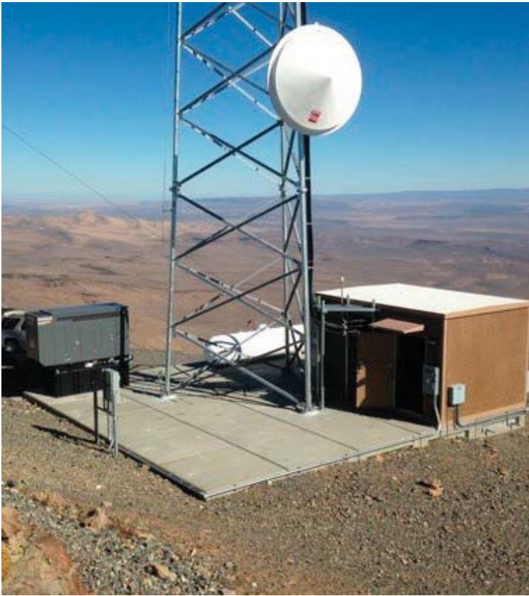
CELL BLOCKS Foundation with wireless cell tower, microwave dishes, antennas, equipment shelter and generator.
