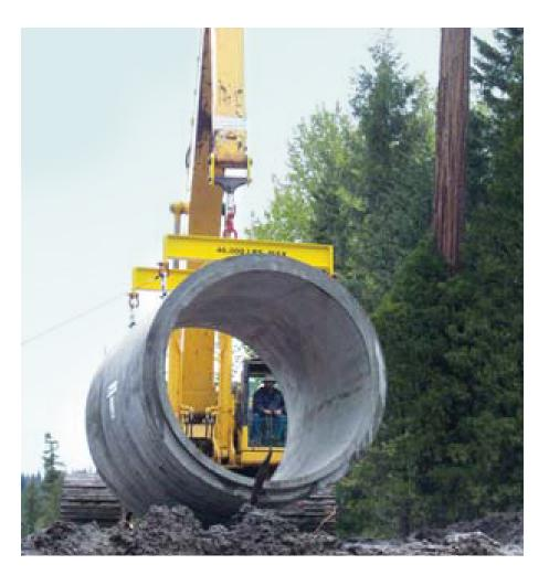
The Lemolo No. 2 tailrace re-routing project consists of in-water construction of the cofferdam for the inlet and an outlet structure. To stay on schedule, they were built from both ends. The 3000 feet of pipe was buried along the Toketee-Rigdon road and across the Toketee recreation area. The pipe will carry 700 cfs from the Lemolo 2 plant tailrace and eliminate ramping in the Lemolo 2 full flow reach of the North Umpqua River.
