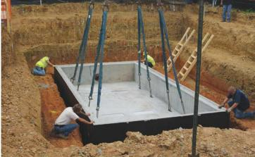
The 102 ton structure was designed in three pieces with a 3 way split slab and separate sump pit. The largest piece was the 37 ton base.
