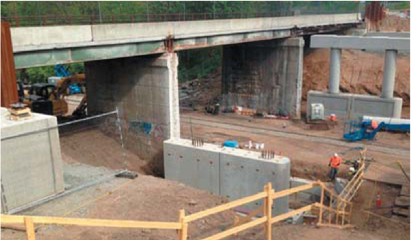
Precast Concrete Bridge - Reconstruction/Rehab
