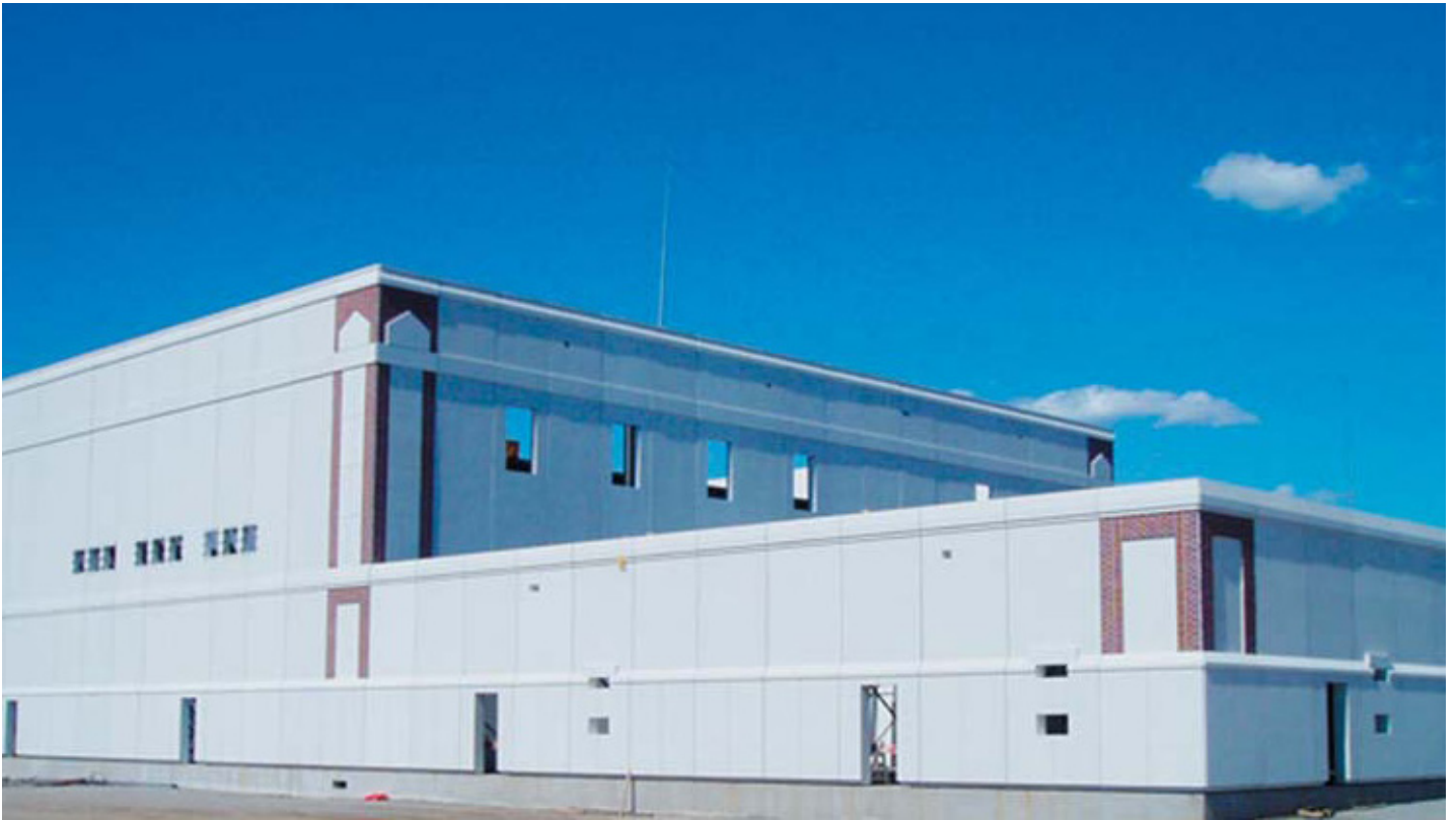
Precast Concrete Gas Insulated Switch Station (GIS) and Control Buildings
