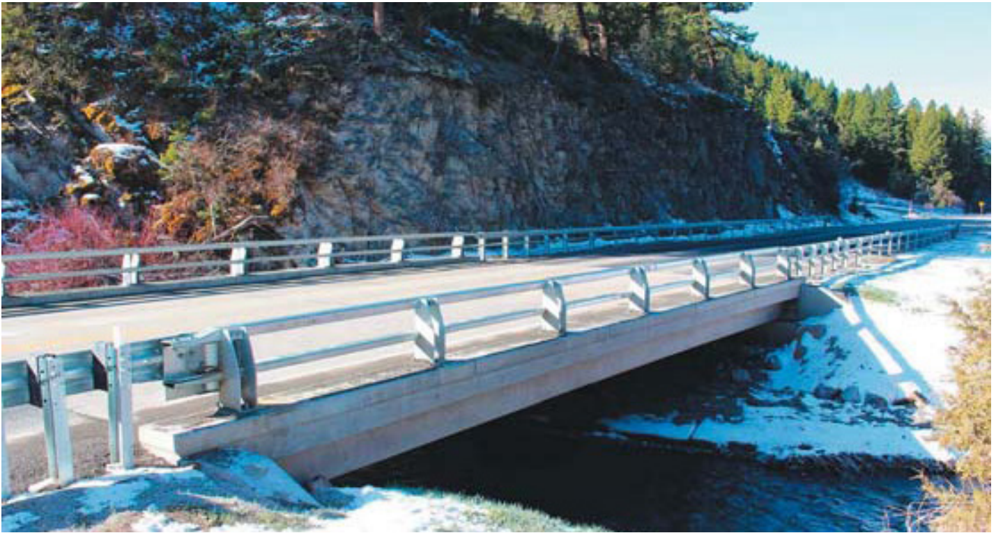
Precast Concrete Bridge Components used for Replacement of Deep Creek Canyon Bridges Using Accelerated Bridge Construction
