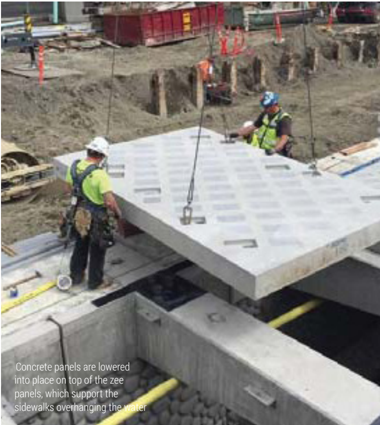
The "Z" Superstructure segments invisibly support the sidewalk from below
