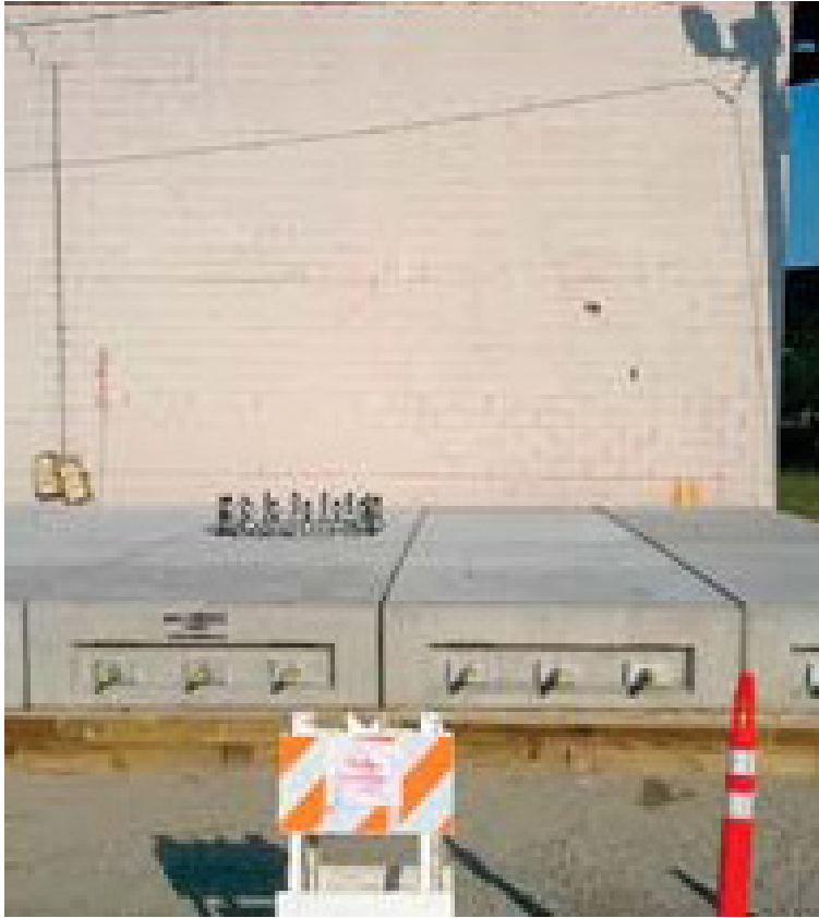
Installation of the CELL BLOCKS onto the wood retaining wall with one-foot of compacted granular material
