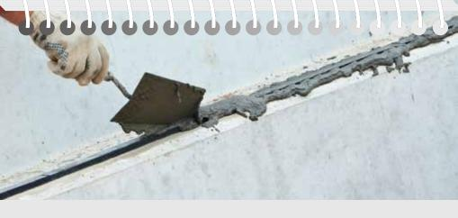
The grouting of hollowcore plank joints is required after install in order to ensure the floor system is fully monolithic.
