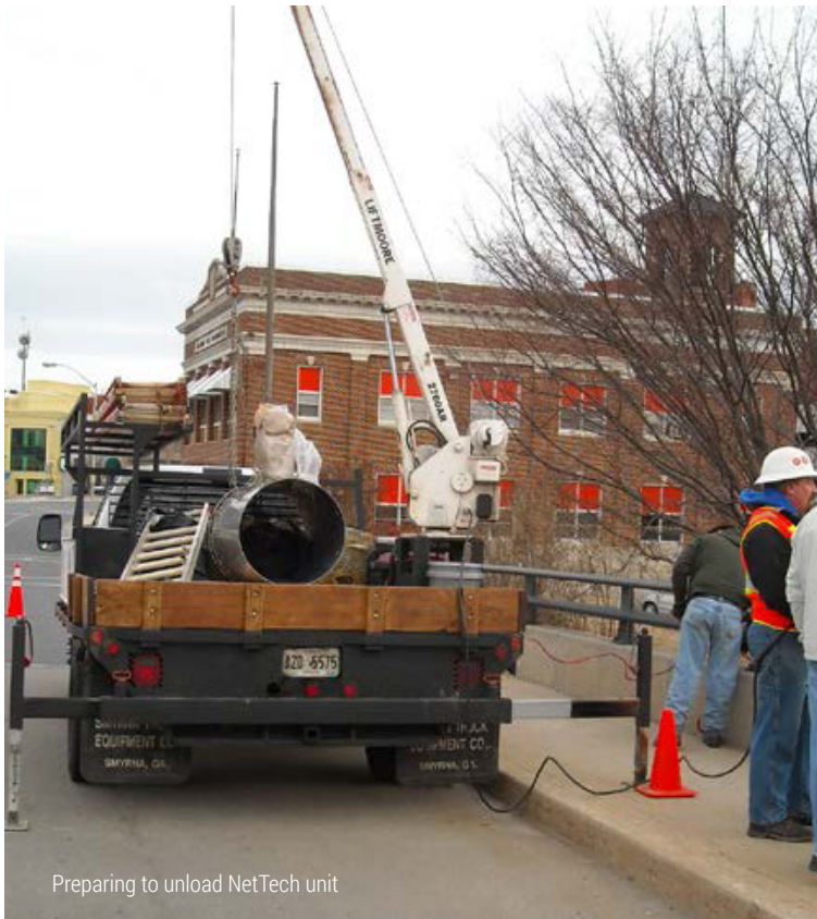
Installation in progress - a boom-lift-vehicle was used to place each NetTech device
