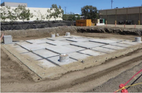
Entire StormCapture system installed and awaiting backfill.
