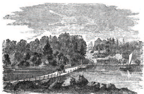
The Floating Bridge across the Schuylkill River was eventually replaced by a permanent bridge in 1838.
