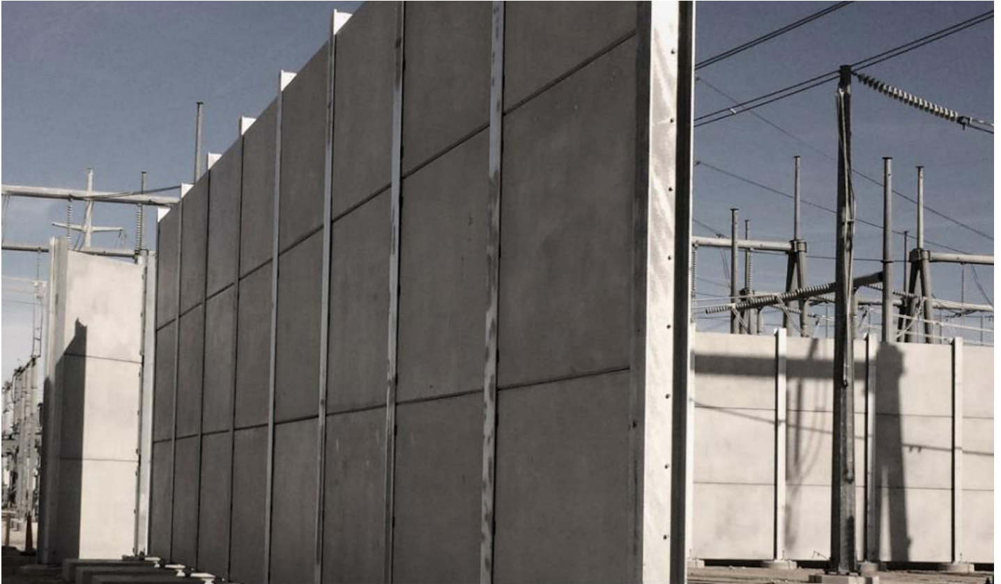
Section of Precast Screen Wall in place outside of the Imperial Valley Substation
