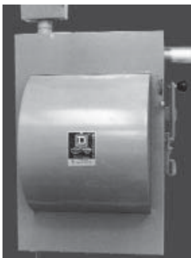
Manual Transfer Switch
