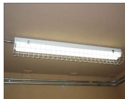
Interior Light with Wire Guards
