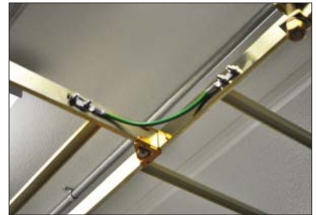
Cable Ladder Junction Tee
