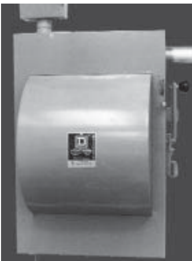
Manual Transfer Switch
