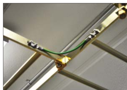
Cable Ladder Junction Tee
