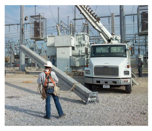
Raise the columns from the storage location using the lift device at the top of the column. Use the rope to guide and stabilize the columns while suspended.
