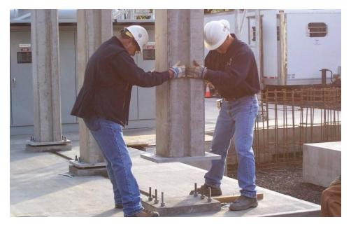
Place the column on the anchor bolts and use the nuts and washers to secure them. Check the columns for plumb in both directions and adjust the leveling nuts to plumb the column. Check the center-to-center spacing of the columns at the bases and the tops to ensure the columns are plumb and adjust as necessary. **Do not apply grout underneath column bases until panel installation is complete in case further adjustments are needed.**
