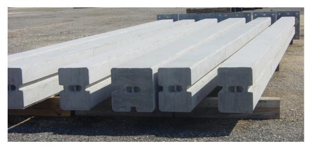
Use dunnage under the column, placed at 1/4 the length from each end, to protect the column during storage.
