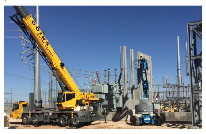
The product weights are shown on the plans. The crane used shall be capable of lifting the product weights at the radius required to pick them off the truck and set them in place on the foundation.
