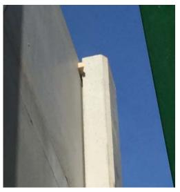
A wooden shim can also be used to assist in inserting the backer rod, using caution not to push it too far into the slot. Cut the backer rod near the column baseplate and repeat for each column slot. Next, fill the column slot with the provided construction adhesive. Use a finger to smooth the adhesive bead.
