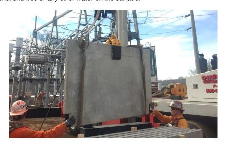
The lifter shall be placed on the centerline of the panel to ensure level picking. The clamp jaws automatically open when all lifting pressure is relieved, therefore, once lifted, do not let the panel rest on the ground or an obstruction as the clamp jaws may inadvertently open. To release the clamp, the operator must relieve lifting pressure on the panel, allowing the clamp jaws to open automatically.
