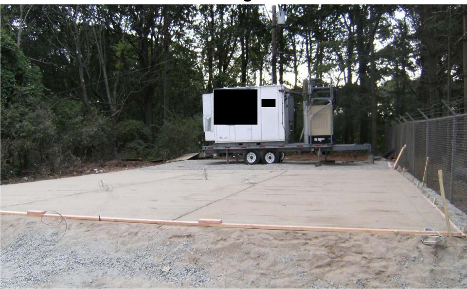
Top ½" to 1" should be concrete sand leveled by using straight screed- Note the screed boards set level on a minimum of two sides
