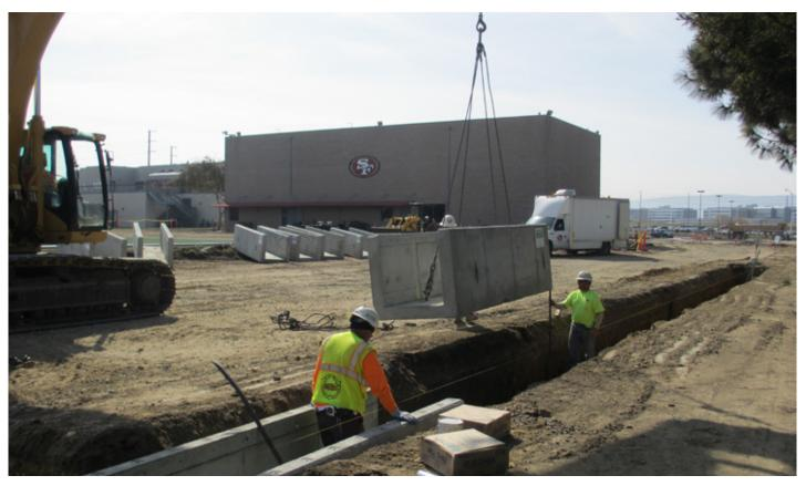
Biofiltration module being installed in the San Francisco 49ers' new stadium complex. The BioMod system collects and treats runoff in the parking lot that will support construction activities. It was on the critical path of site development, before virtually any other construction could begin, so there was heavy time pressure to produce and install the system.
