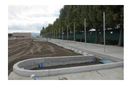
These special wide modules were custom designed and fabricated for the 49ers project. They are needed to increase surface area of the filtration system to compensate for site conditions. Each drains 7,500-10,000 sf of parking lot. Custom fabrication did not delay the tight production schedule for this system.
