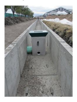
The second system in the east parking lot of the stadium included an overflow drain with a unique filter device that retains floatables within the system, seen here before being piped and filled with filtration media. any production delays or presented any problem to fit into the modular system.
