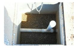
Looking down into the empty unit, the drainage pipe is installed and the BioPod is ready to receive a tree and be filled with planting/ filtration medium.
