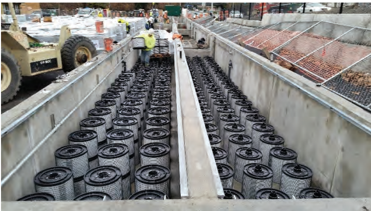
Redmond Regional Water Treatment Facility, Redmond, WA
