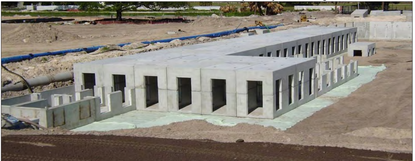
StormCapture System During Installation Process
