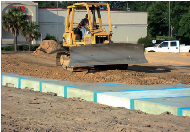
StormCapture modules are designed for HS20 traffic loading.
