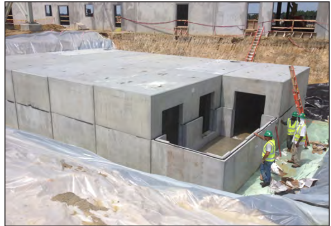
StormCapture detention system installed beneath office parking lot.
