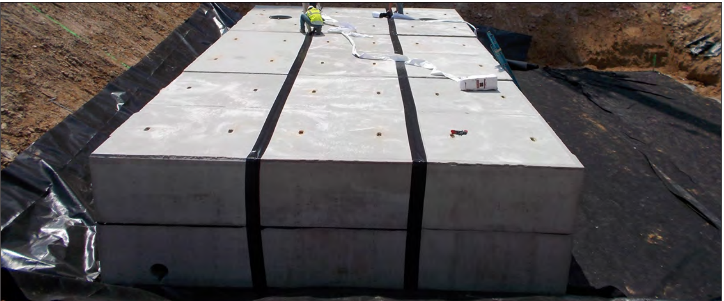
Sealed Joints Between Modules
