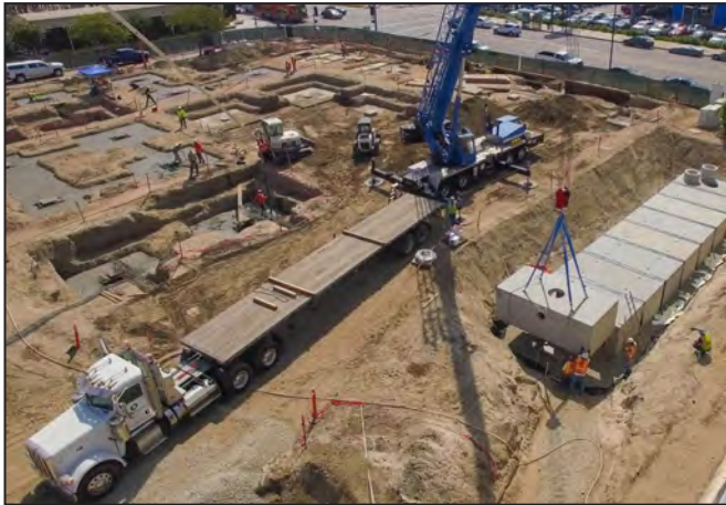
Same-day staging and installation of StormCapture project.
