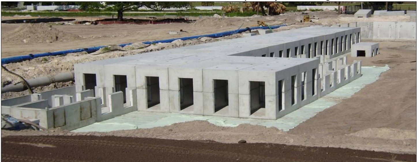
StormCapture System During Installation Process
