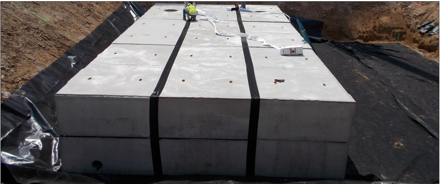
Sealed Joints Between Modules
