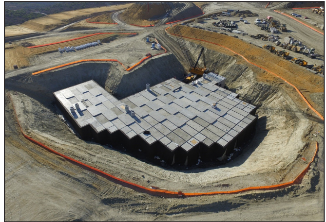
StormCapture offers fast installation with minimal handling.
