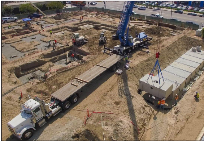
Same-day staging and installation of StormCapture project.
