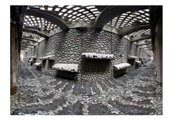
precast light penetrating sidewalk panels to promote and improve marine habitat underneath the 3,500-foot structure.
