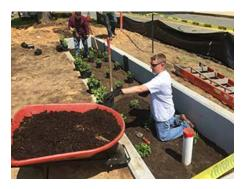
Oldcastle Precast's Edgewood, Md. and Fredericksburg, Va. facilities provided two atgrade precast concrete bio-retention planters and one above-grade planter designed to capture, retain and filter stormwater runoff. A 4-foot by 24-foot by 16-foot bio-retention planter was created near Parking Lot #20 to collect runoff from the street and parking areas. The run-off was diverted to the retention system by means of a parking lot channel created by the site contractor.
