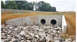
As a part of the roadway improvements, PADOT required contributory stormwater management systems to accommodate increased roadway stormwater run-off from the new facility. This portion of the project required Oldcastle Precast to produce an additional 2,322-feet of RCP pipe, 14-inch to 23-inch elliptical pipe and 18-inch to 48-inch diameter round pipe, catch basin inlets with bike safe grates, headwalls and manholes.
