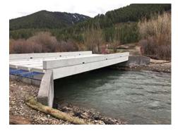
The new bridge was designed with a span of 45-feet. Due to this span length, not being conducive to standard precast slabs, Oldcastle Precast engineers partnered with VSL Structural Technologies to create a custom precast solution. Oldcastle Precast and VSL decided to install post tension cables in the slab during the precasting process.
