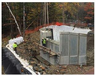
The use of precast concrete bridge components allowed for the rapid construction of the bridge substructure. The bridge abutments were delivered, installed, and grouted over a 2-day span.
