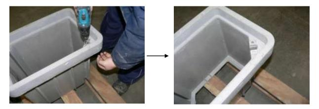
2. Then take the top box and drill one hole on each of the ribs under the hardware at 3" from the bottom.
