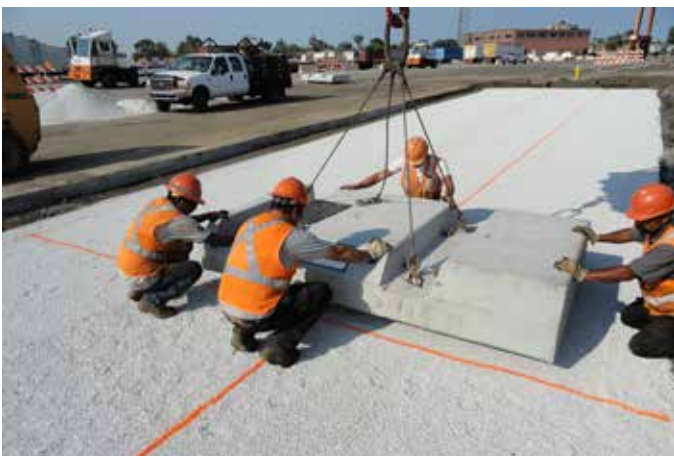
Placing StarTrack HD Module
