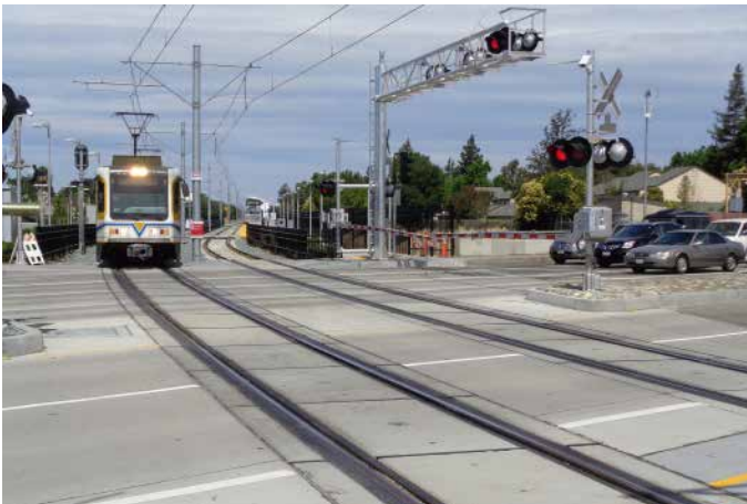
Light Rail Crossing
