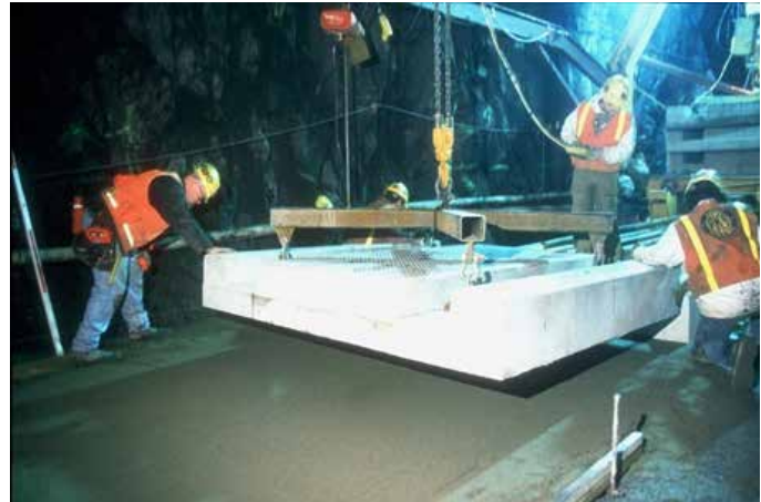
Placing 7.5 TF StarTrack Module
