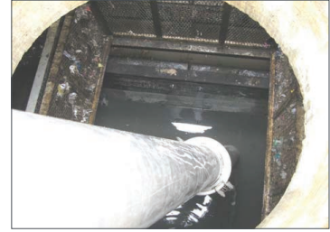
Open lower screen panels to remove sediments via vacuum truck.
