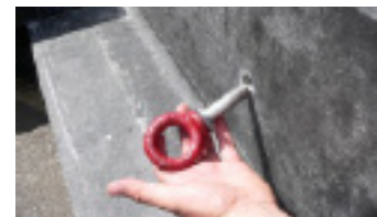
3. Insert eye bolt with eye toward inside of channel
