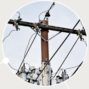
Existing wiring can be left in place, no need to transfer telephone, CATV, or fire on joint-use poles.
