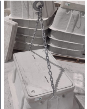
Use correct strap/chain length to ensure proper angle.
