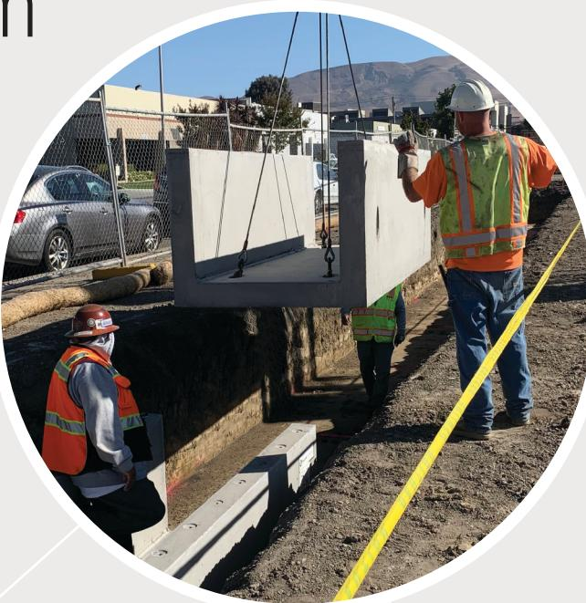
Efficient integration of bioretention in tight sidewalk applications.
