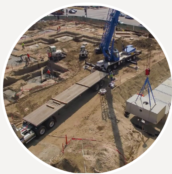
Same-day staging and installation.
