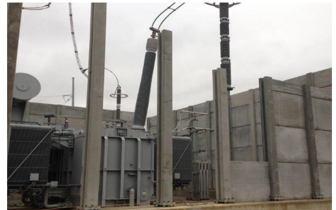
Follow drawings to ensure panels are in correct location
