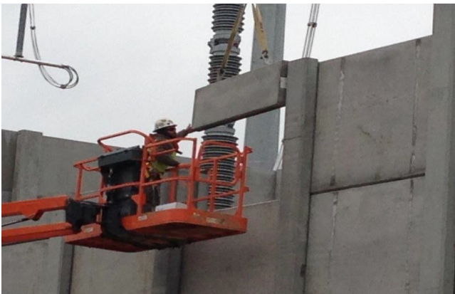
Continue setting panels and ensure no gaps between panels
