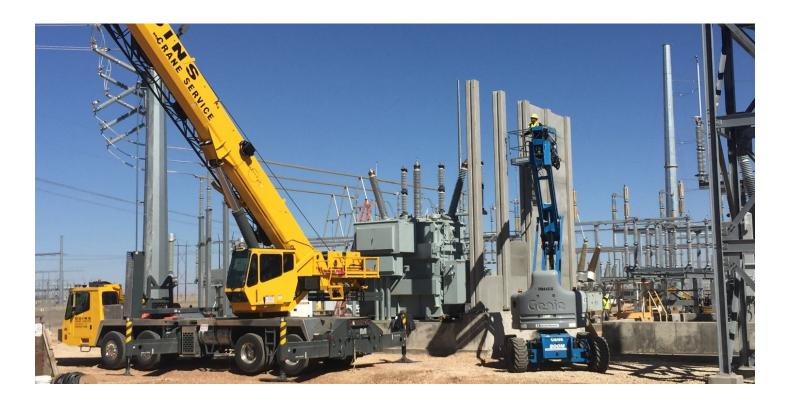
The site conditions and access points will determine the placement of the Crane, Personnel Lift, and Truck egress to allow the TruFireWalls™ to be installed. A typical TruFireWalls™ will include all components on one truck. Larger walls will require additional trucks.
