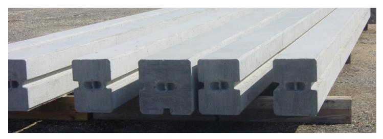
Use dunnage under the column, placed at 1/4 the length from each end, to protect the column during storage.
