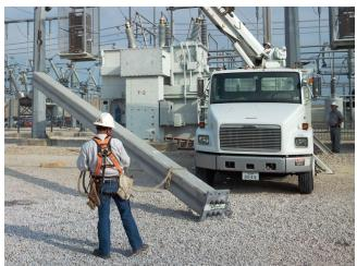
Place the column on the anchor bolts and use the nuts and washers to secure them. Check the columns for plumb in both directions and adjust the leveling nuts to plumb the column. Check the center-to-center spacing of the columns at the bases and the tops to ensure the columns are plumb and adjust as necessary. Do not apply grout underneath column bases until panel installation is complete in case further adjustments are needed.
