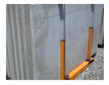
The panel clamp shall remain with the owner to allow disassembly of the TruFireWalls™ in the future.
