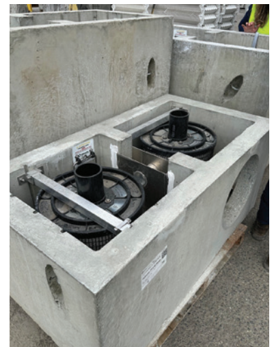
Cartridge placement with hold down bar
