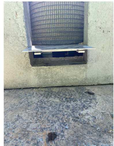
Field joint plate in position
