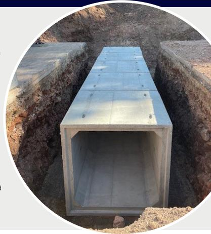
The project presented several critical challenges. To begin with, a swift turnaround was essential, with the detour needing completion in under 15 days to minimize disruption and restore this vital transportation route. Logistically, transporting 120-feet worth of box culvert from Oldcastle's Nampa, Idaho, plant to the project site required meticulous planning and coordination due to the distance and logistical constraints.
