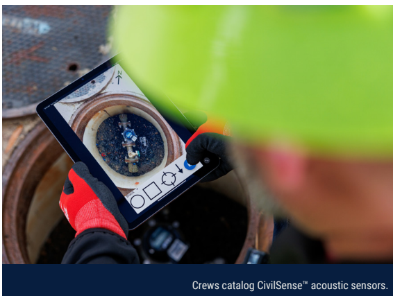
Advanced acoustic sensors are installed in targeted areas.
