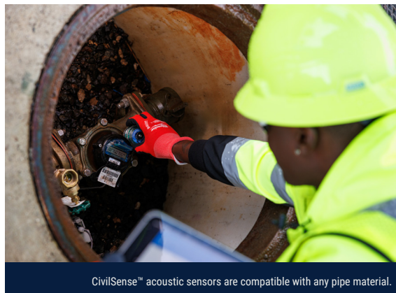
Advanced acoustic sensors are installed in targeted areas.
