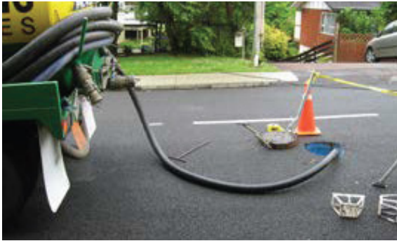
Figure 2: Sediment is removed from the sump with a vactor hose. Confined space entry is not required for this step.
